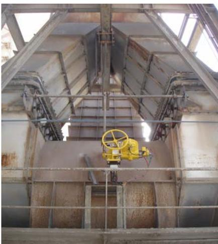
Rack & Pinion actuators are complex units. Continuous and uneven (due to piston offset) gear tooth wear reduces the unit life. Carbon steel springs on spring return units become corroded. All this leads to a lifetime of only up to 1 million cycles, although many units may fail to reach this figure in a harsh cement plant environment.
